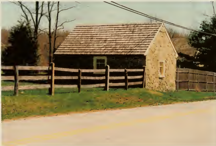
Photograph #23: A serpentine carriage or wagon house, now a garage, in Westtown Township. The serpentine came from the Serpentine Ridge Quarry, located nearby.
